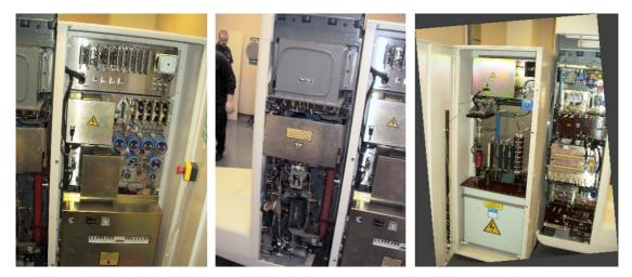
The accelerator power circuits (left), the pulsing circuits (middle) and the modulator and focus supplies (right). John Draper is in the background of the middle image, wandering, along with everyone else, how not to get roped in to this project.
